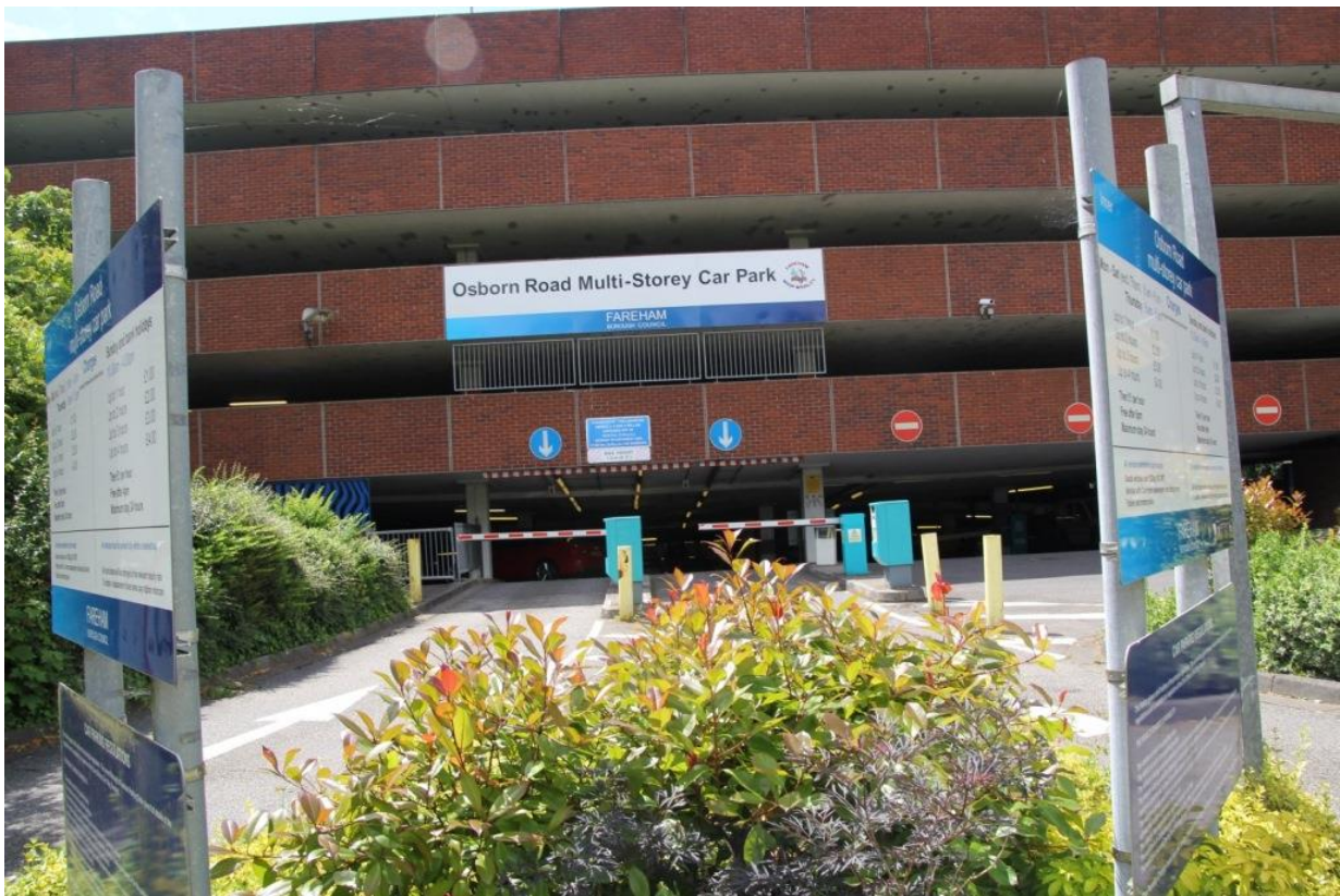
Osborn Road Multi-Story Car Park
