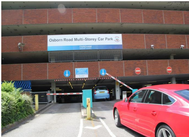
Osborn Road multi-storey
